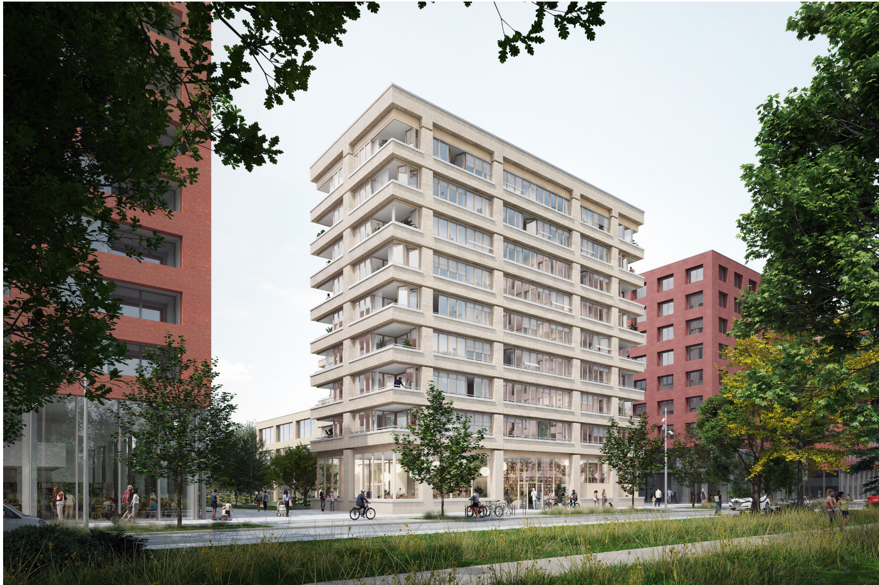
LIONES DEBS ARCHITECTES STARLETTE HOUSING STRASBOURG, 2022
