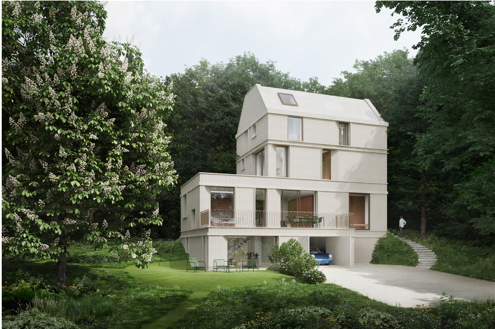
FRANCOIS CHAPPELLE ARCHITECTS DILBEK HOUSE DILBEK, 2022
